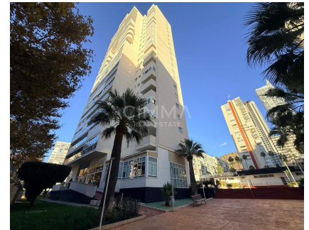
Ascensor, All exterior,
